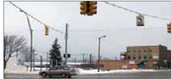
Existing Condition C. DeChiaro
